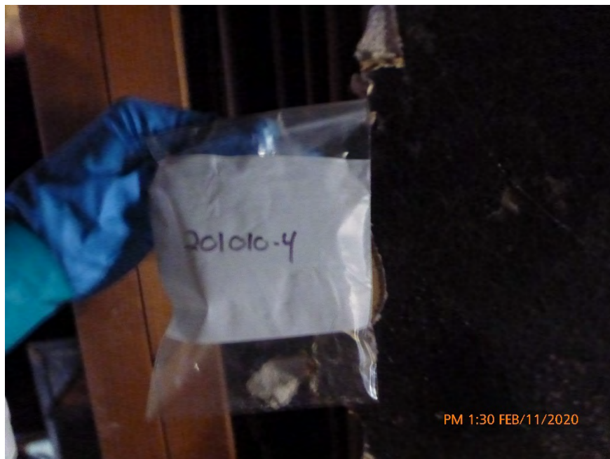
Photograph 10: February 11, 2020, at approximately 1:30 PM - View of Sample #201010-4 obtained from the material depicted in Photograph #9.
