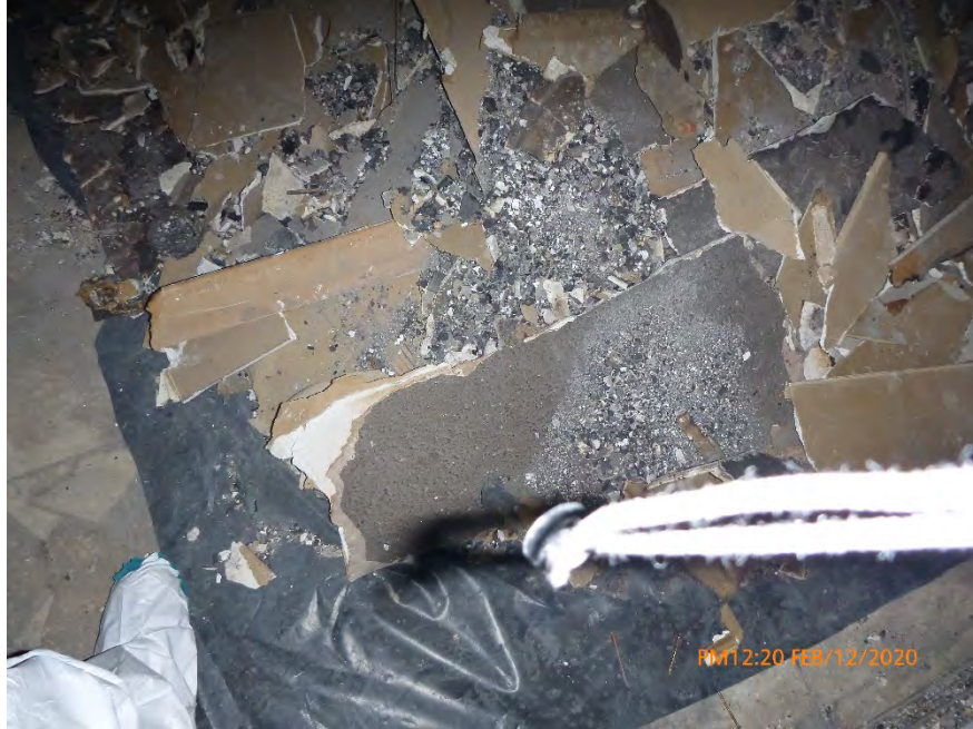
Photograph 25: February 12, 2020, at approximately 12:20 PM - View of textured drywall in a debris pile inside the north room of Unit 3. The material was sampled and later determined to contain 3% Chrysotile Asbestos by the point count method using polarized light microscopy. The material was in a dry condition with no evidence of moisture.
