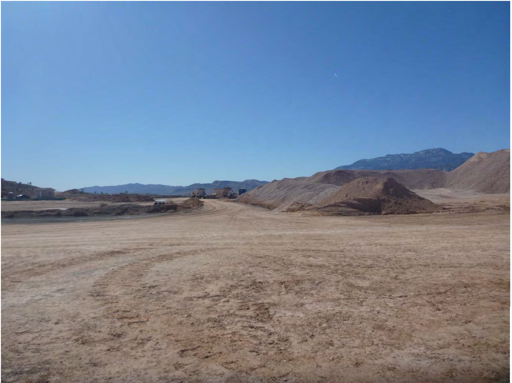
Photograph 16- Gypsum Paved Haul Road; on-site (EU: B02) shown as unpaved. Photograph by Camon Liddell.
