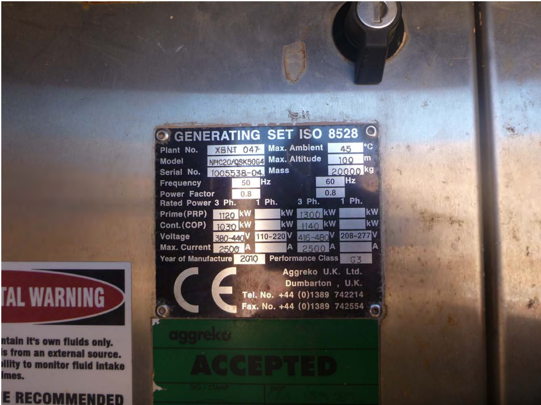
Photograph 8- Serial plate of Continuous Duty Diesel Engine (Generator) (EU: C01) [Crusher] depicting a 1,300 kW rating. Photograph by Canon Liddell.
