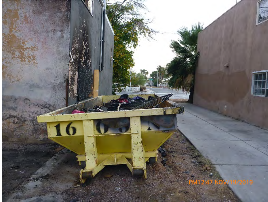
Photograph 22: November 19, 2019, at approximately 12:47 PM - View of the 16 cubic yard dumpster which contains ACWM. The dumpster remains uncovered.
