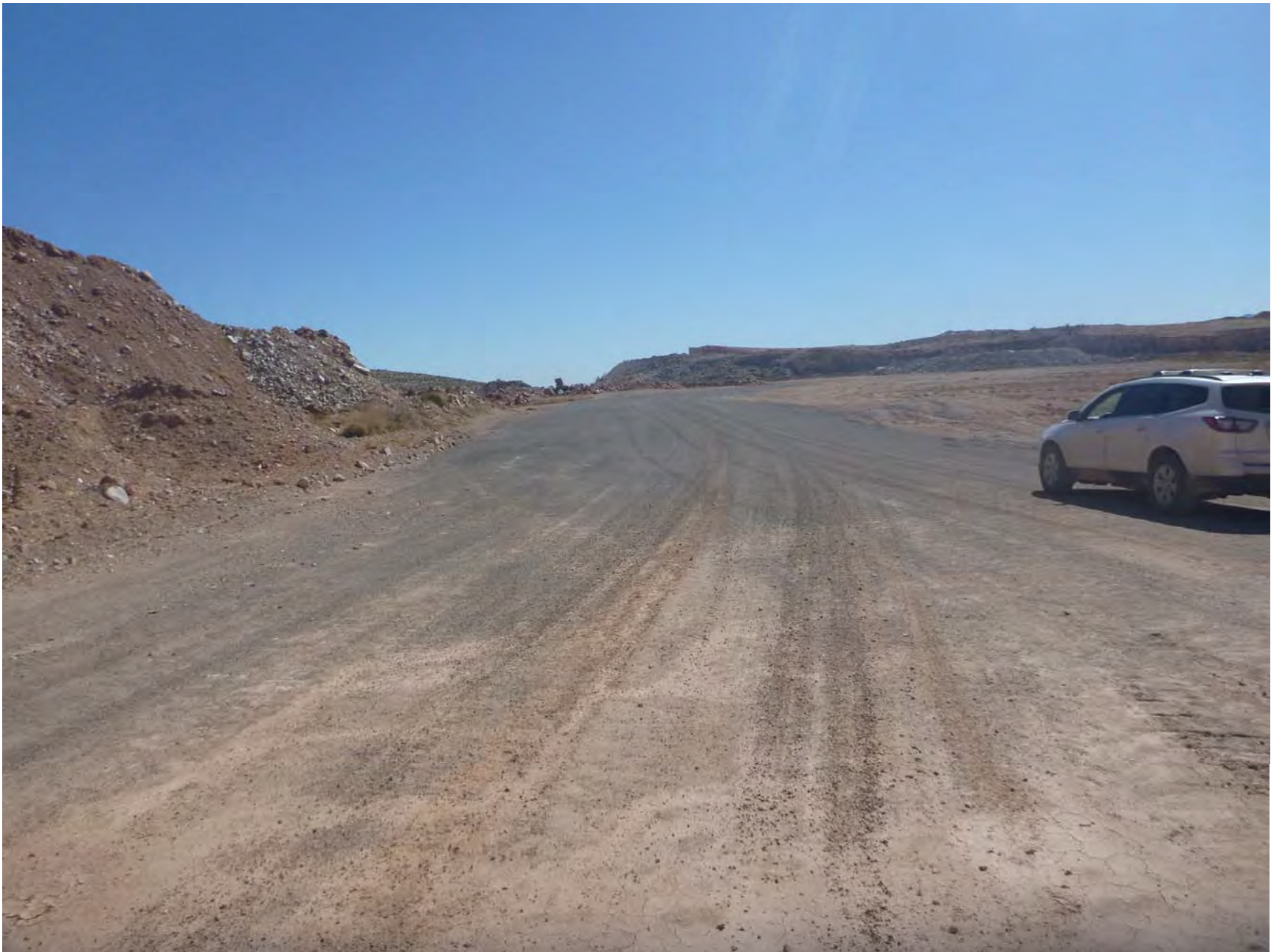
Photograph 18- Gypsum Paved Haul Road; Overburden (EU: B03) shown as unpaved. Photograph by Camon Liddell.
