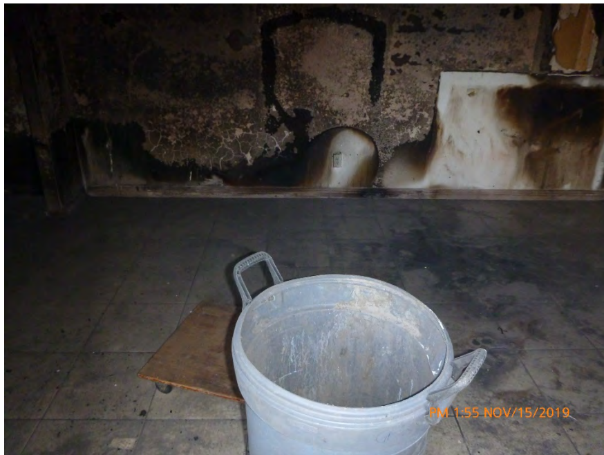
Photograph 6: November 15, 2019, at approximately 1:55 PM - View of a waste bin in the north room (Master Bedroom) of Unit 1. Note the lack of a significant amount of debris on the floor.
